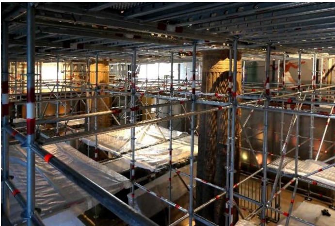
Fig. 1 Scaffolding in the public gallery. (© Markus Krön)
