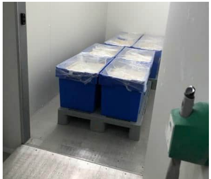
Fig. 2 The entrance to the professional cold storage cell. (© Tykwer)
