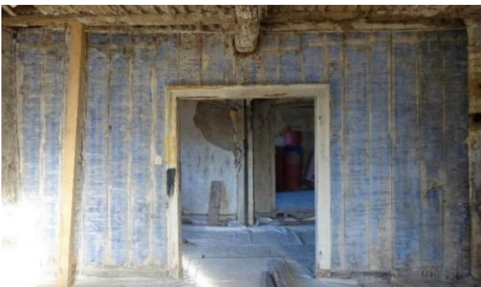
Fig. 1 Overview room partition with wallpaper. (© Christian Hartwig)
